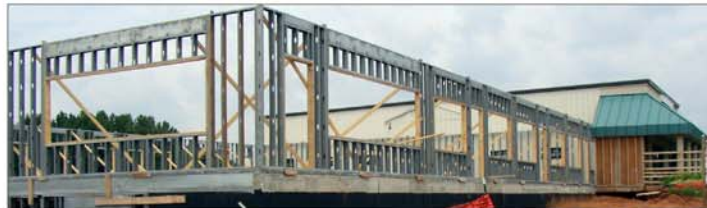
Lakewood Professional Center Deck Addition
